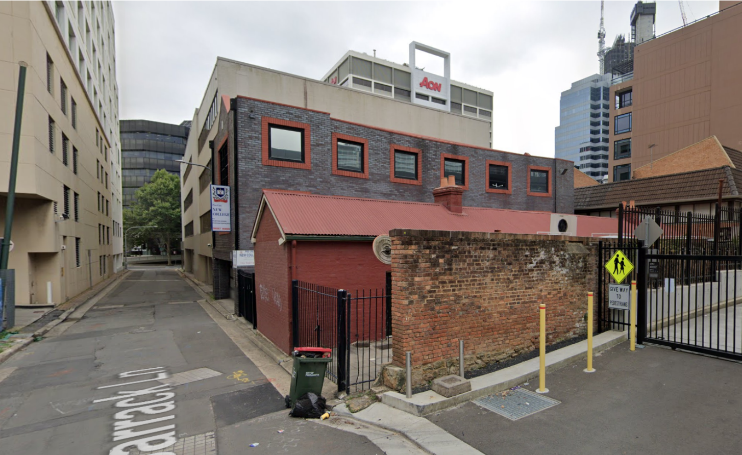
View 1 - 3 Barrack Lane and Convict Wall
