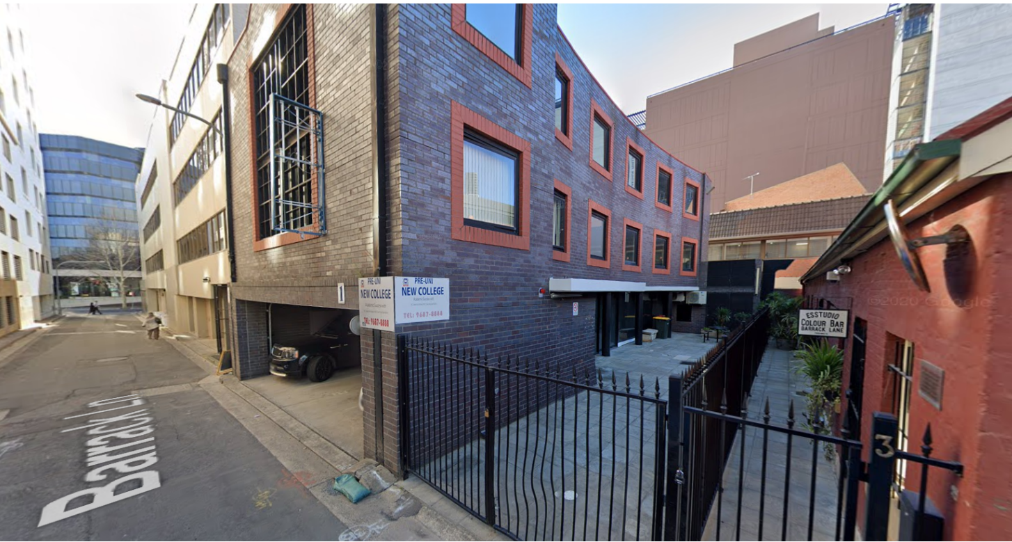
View 3 - 1 and 3 Barrack Lane
